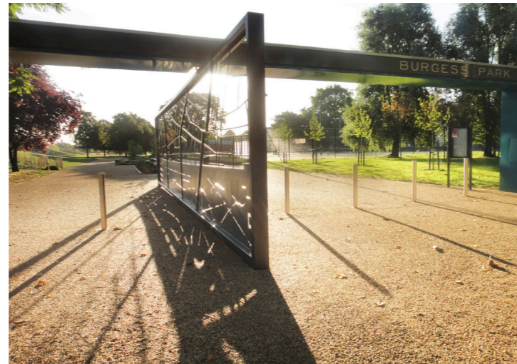
EXISTING PRIMARY ENTRANCE (CAMBERWELL RD)
