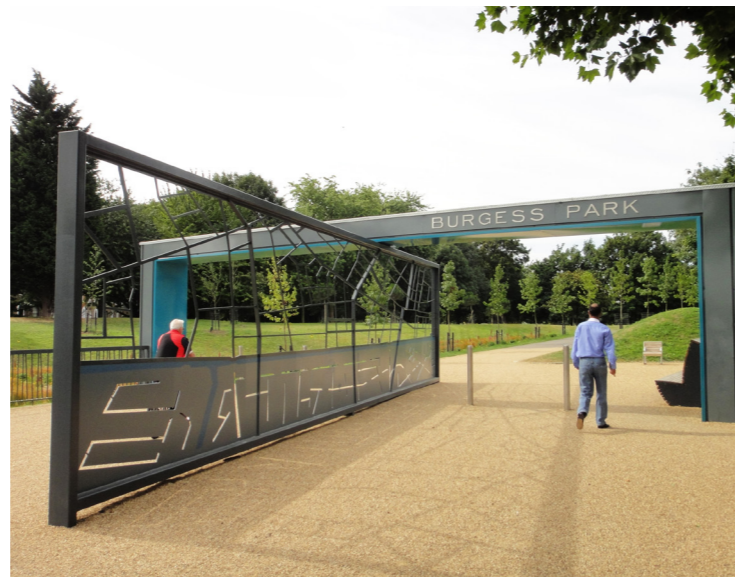
EXISTING PRIMARY ENTRANCE (OLD KENT ROAD)
